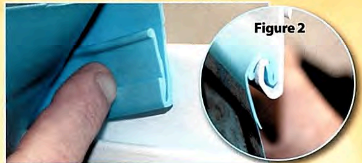
When your pool has a standard bead track, use the EZ Bead to slip right into the channel at the top of the pool wall. (Fig 2)
